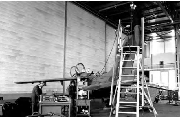
Figure 3 : Early investigations of radio-electric disturbances on an A.M.D. Alpha-jet
