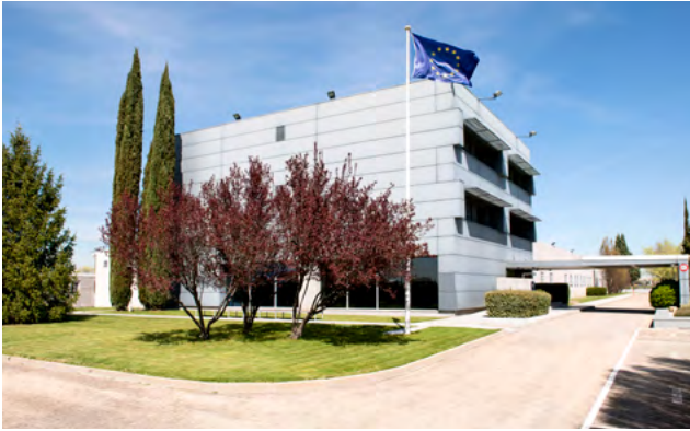
SatCen building, ©SatCen
